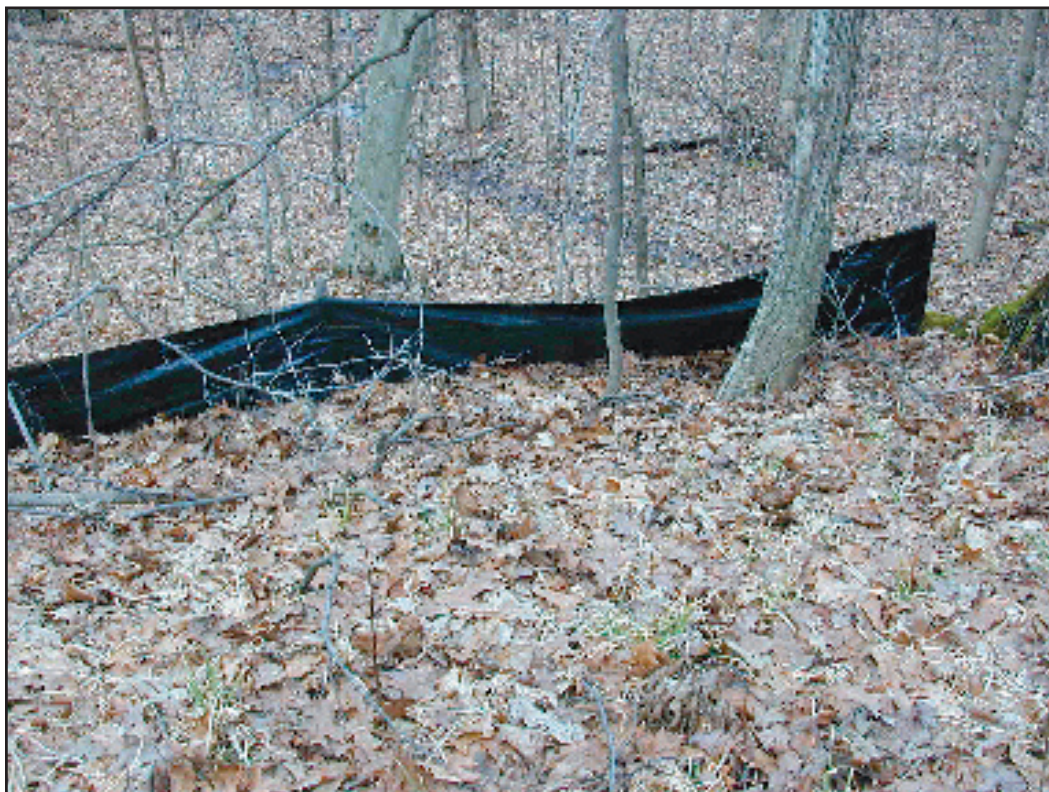
Figure 7. Effective application of silt fence.
