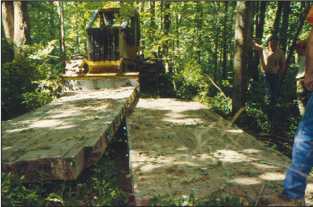
Figure 22A. Portable logging bridge installed with skidder.
