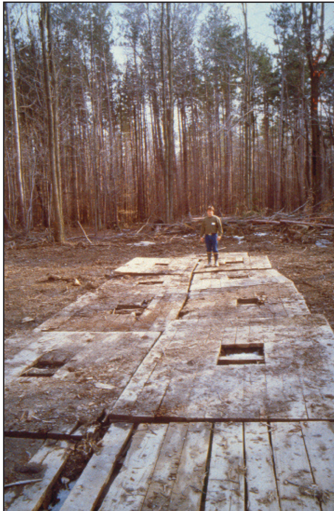
Figure 16. Protective wooden mud mats.
