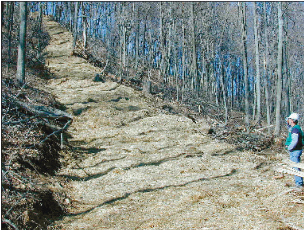
Figure 27. Properly installed mulch on new seeding.
