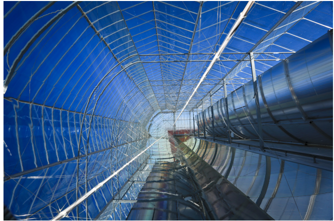
Fig. 1.3 View from inside the enclosed-trough parabolic solar mirrors, used to concentrate sun and generate steam for enhanced oil recovery (EOR).
