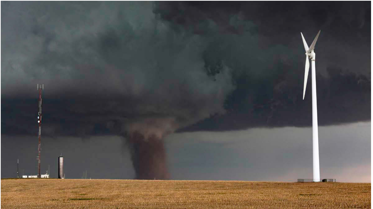
Figure 1. Power infrastructure faces a variety of natural threats that can cause damage and disrupt the power system. Designing and siting power systems to minimize impacts from threats is important. Photo from iStockphoto, 531920932
