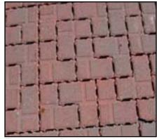
Figure 2.11.7 Pervious Interlocking Concrete Pavement
